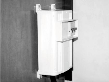
A ground fault circuit interrupter (main switch) protects the electrical system of the motor home.
