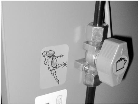
Fig. 66: Quick-closing valves
