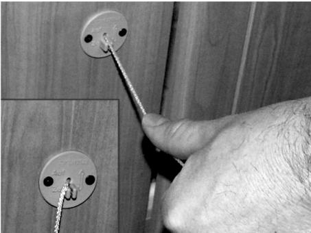
Fig. 73: String-operated baffle
