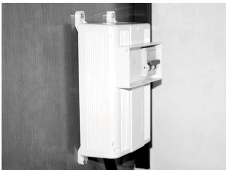
Fig. 57: Ground fault circuit interrupter (GFCI)
