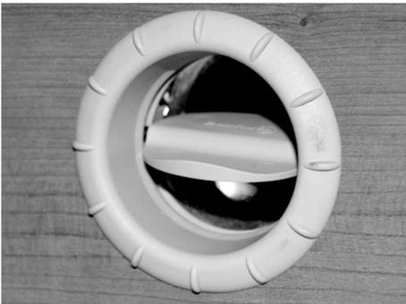
Fig. 72: Hot-air nozzle, open
